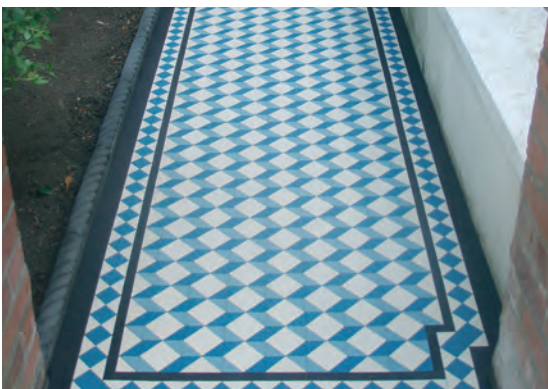
Photograph courtesy of Tiled Perfection
